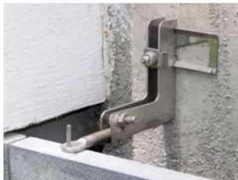
Figure 4 Natural stone with anchor
