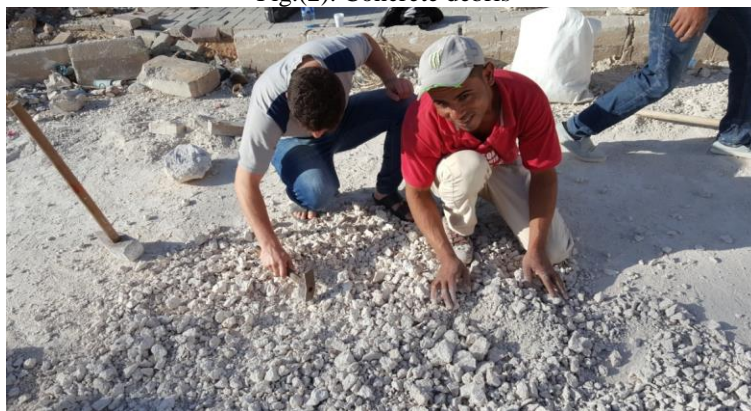
Fig.(3). Crushing of Concrete debris
