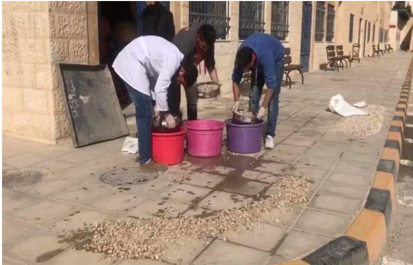
Fig.(7). washing and drying of aggregates
