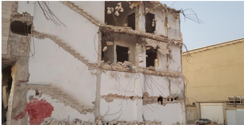
Fig.(1). Old demolished buildings
