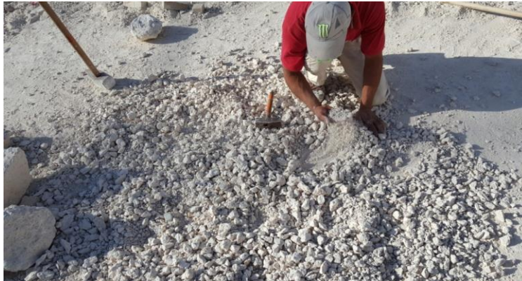
Fig. (4). collecting of small concrete pieces
